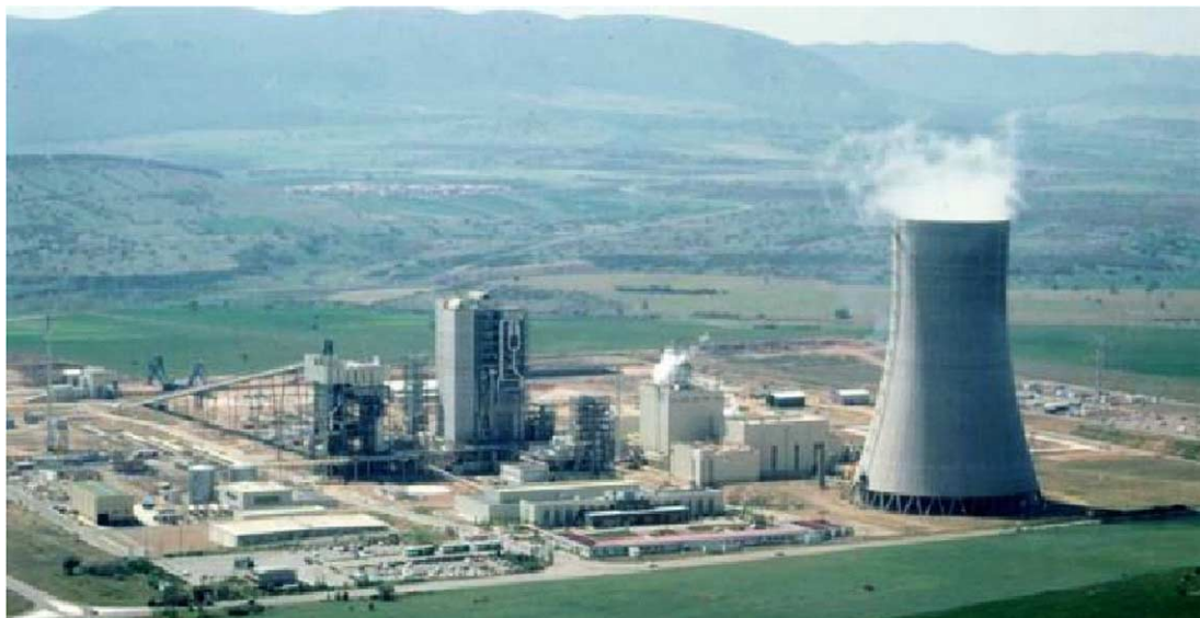
Fig. 5. ELCOGAS 335 MW e IGCC plant at Puertollano, Spain.
